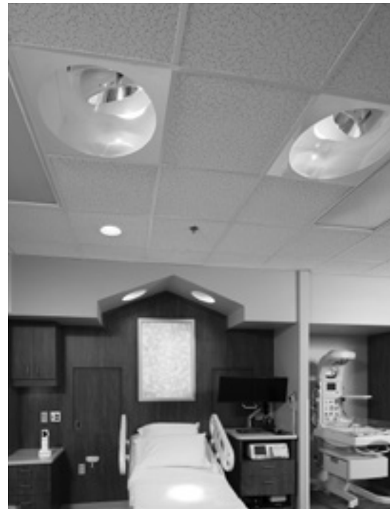
Sample of installed ceiling mount lights with wall control and wand
